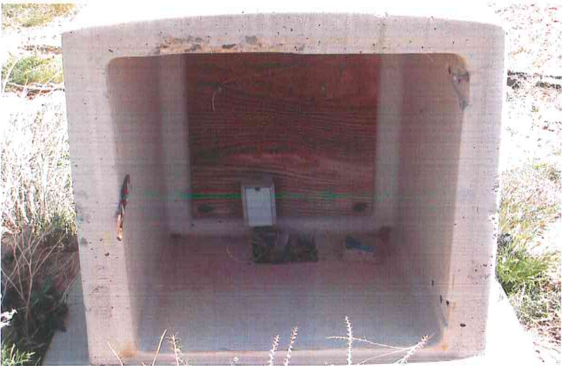
No. 38 – Electrical outlet inside the concrete casing.
