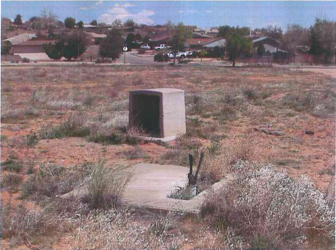
No. 37 – Concrete encasement / utilities pad which has been abandoned.
