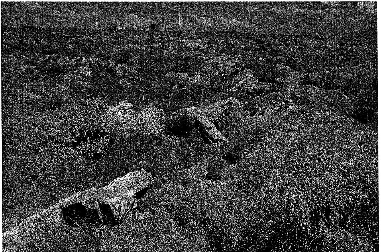
Concrete and surface debris along the arroyo in the northwest portion of the site
